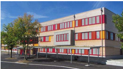
Gymnasium Sonthofen 2 Accublocs, total 23'250m 3 /h
