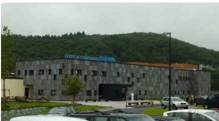
Lahn-Dill-Bergland Therme, Bad Endbach 1 Accubloc, total 5'001m 3 /h
