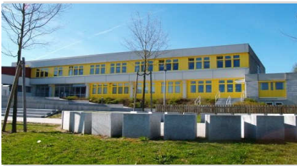
Realschule Au, Hallertau 2 Accublocs, total 11'040m 3 /h
