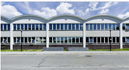
Pausa Tonnenhalle, Mössingen 2 Accubloc, total 4'928m 3 /h
