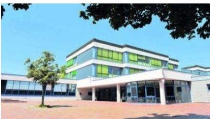
Schulzentrum Landsberg 2 Accublocs, total 10'800m 3 /h
